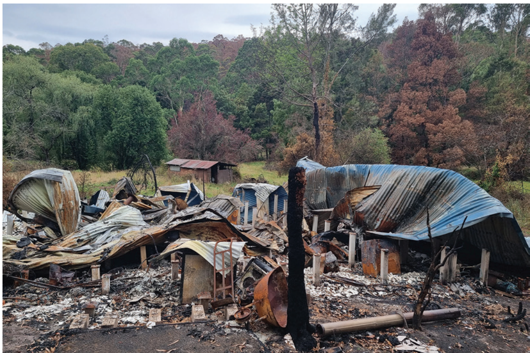
A fire damaged building in Gellibrand.
