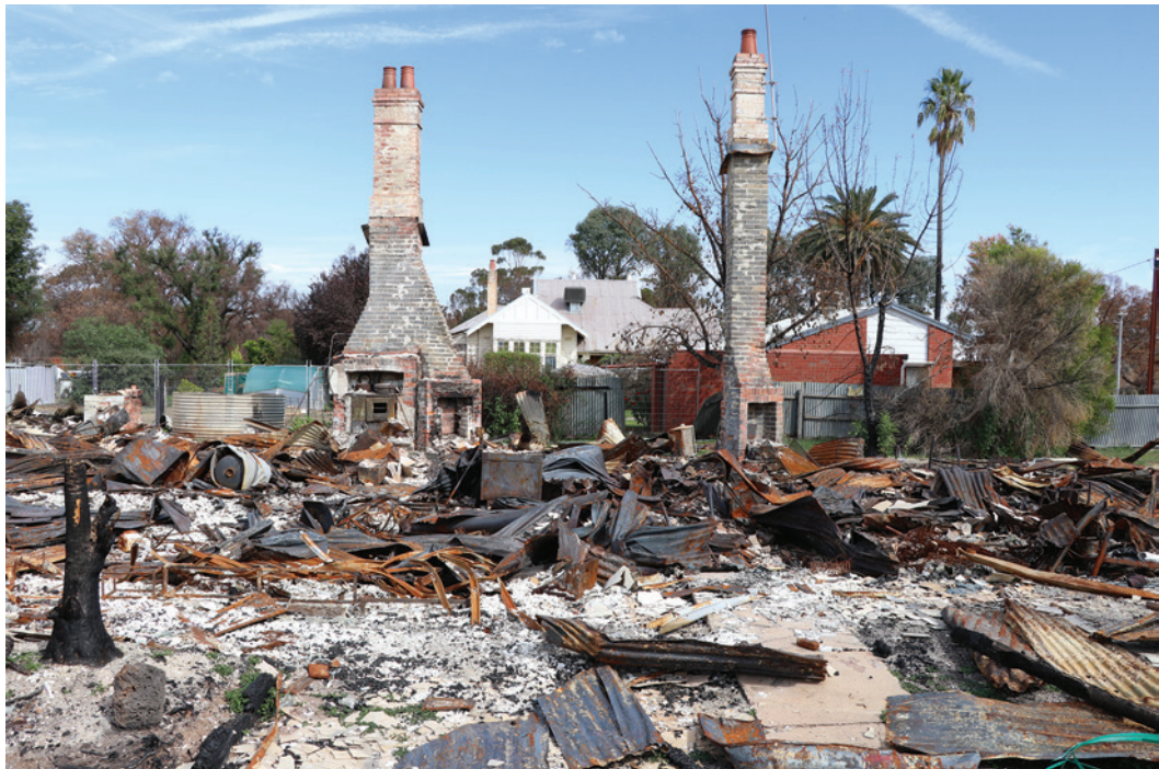
A fire damaged building in Natimuk.
